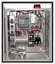
These open face control panels provide complete management of the integrated "Perc-Rite® Drip Dispersal System". The control includes manual override capability bypassing the PLC, automatic field flushing, and multi-zone Control. The build in sceen has many built in options best operator control.
